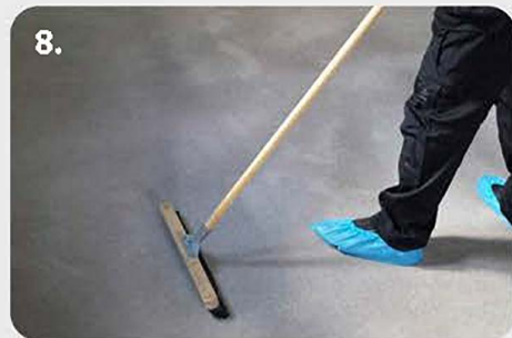
8. Set pile - Lay fibres flat to speed drying.
